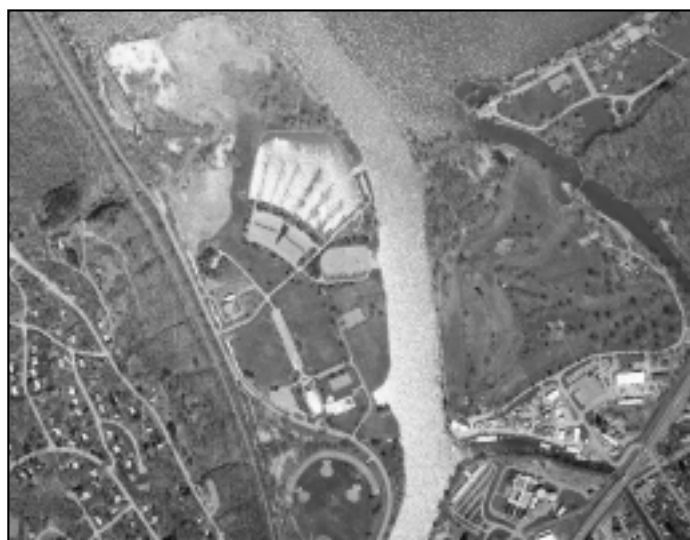
The Ithaca Area Waste Water Treatment Facility (IAWWTF) would process the hydrolysate byproduct from the Veterinary College using both anaerobic digestion and aerobic treatment processes. The treatment co-generates electricity and heat, used at the IAWWTF (lower right corner, look for two circles close together).
