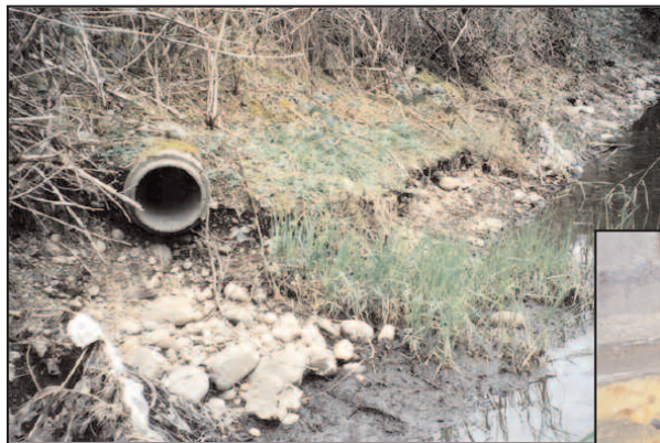
“Outfall” is the name given to pipes such as this one that drain directly to a creek.
