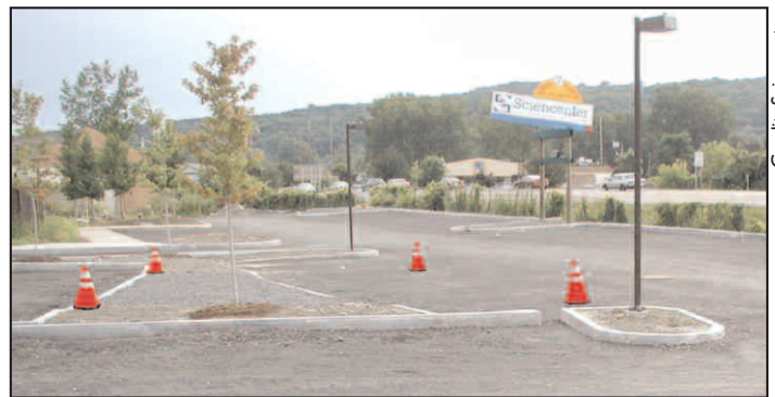
The four cones mark the corners of the underground infiltration basin.
