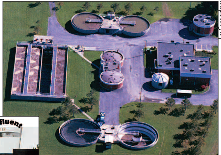
Wastewater treatment plants provide vital service but take energy. Four percent of the nation's electricity use goes to moving and treating water and wastewater, according to the University of Michigan's Center for Sustainable Systems.
